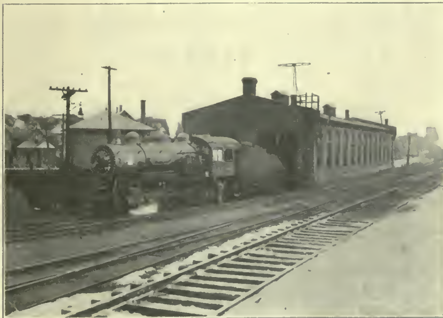
FIG. 679. FACILITIES TO BE REMODELED. Present steam locomotive engine house of the Chicago Short Line Railway, which will be retained without change, for the care of electric locomotives.
